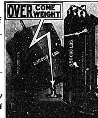
The Floors Won't Sag From Compressed Air Ballast
